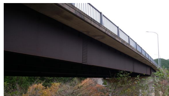
Fig. 1: Show the Toyokuni bridge overview
