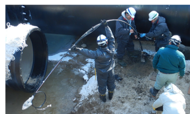
Fig.1 層別沈下計の設置状況 Installation status of stratified subsidence meter
