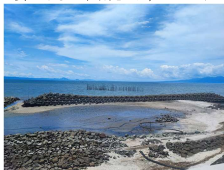
Fig. 1 Settlement phenomenon of tetrapod on soft clay ground
