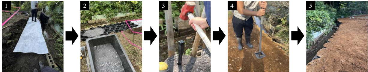
Fig 1 Construction procedure of geocell
